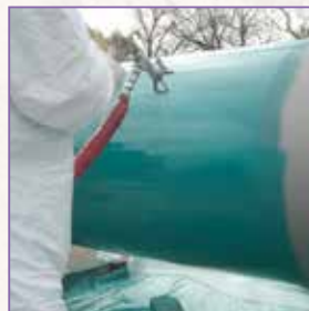
Corrosion prevention of new pipelines
